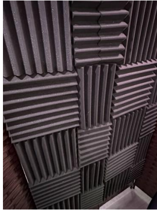
Above: acoustic foam is often used in recording studios to reduce echoes.
